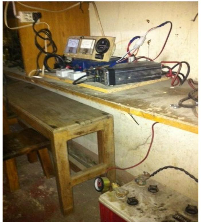
For short brown-outs, this is the 3-year old existing solution, a fully automatic battery-inverter transfer switch that carries selected lights, TV, fans & internet modem. Complete circuit and ladder diagram is below.
