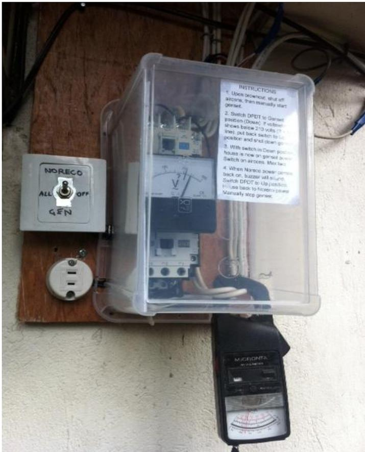
Contactors and wiring are protected by Tupperware box.
