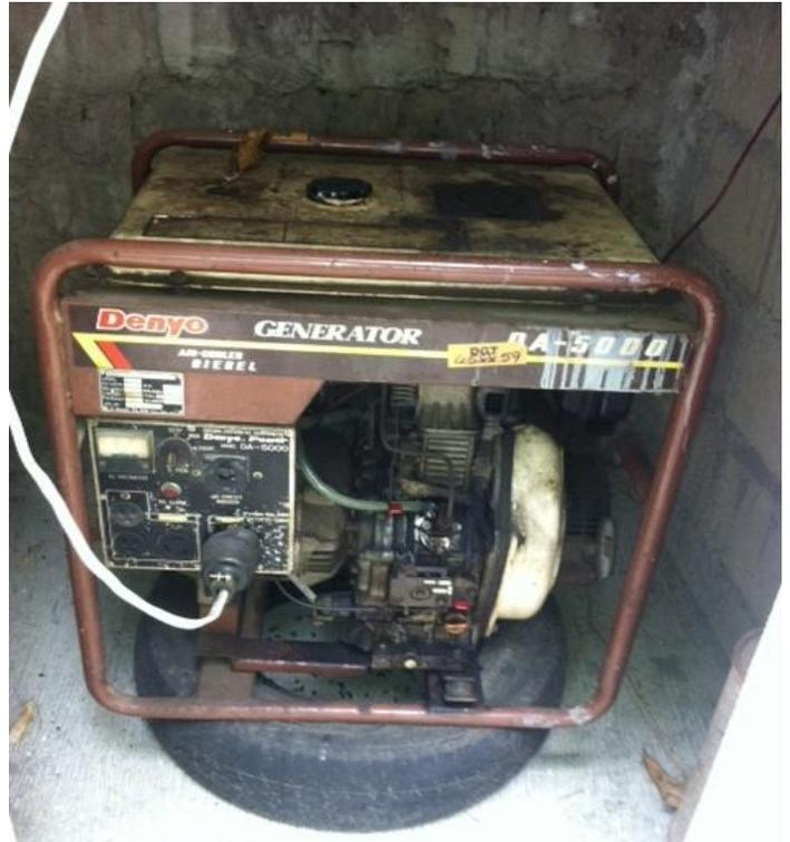
Inside shed is electric-start diesel generator (5 kw)
