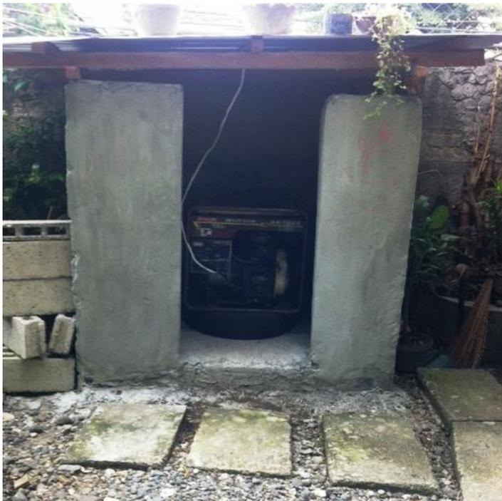
Generator shed. Next project is to try to noise-proof the structure to minimize the racket, by perhaps lining it with styro-por and putting a louvered door. Generator is air-cooled.
