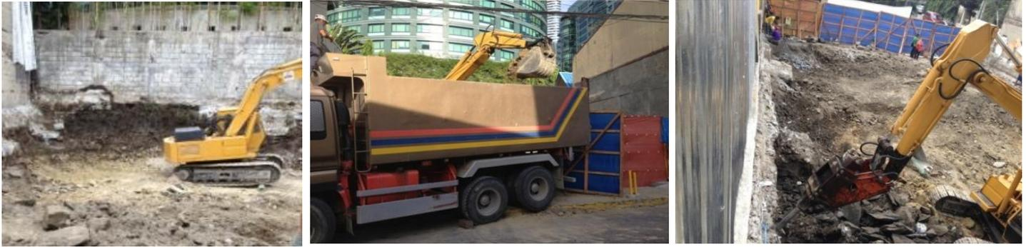
The culprit was a backhoe tractor with an articulated arm that is fitted with bucket to scoop up and load debris on trucks such in the middle photo, or a powerful hydraulic jackhammer that thumps it's way into the concrete structure to break it up, or into the adobe bedrock to dig one level below grade for the underground garage, as in the right photo.
