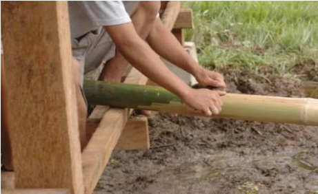
Most laborious part, scraping clean the bamboo, then halving it for walls.
