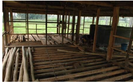
More floor joists, and concrete T&B
