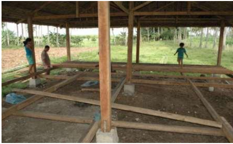
After posts and roof, floor was next.
