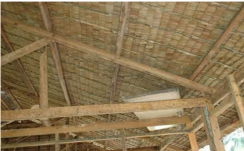
View of ceiling early in construction.
