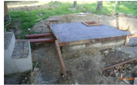
Partly complete septic tank with steps to back entrance shown.
