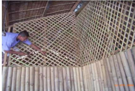
View after interior walls are put up.
