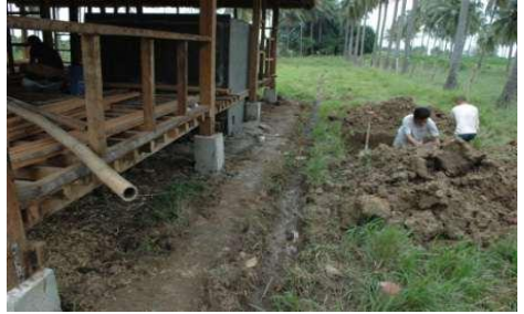
Digging the septic tank
