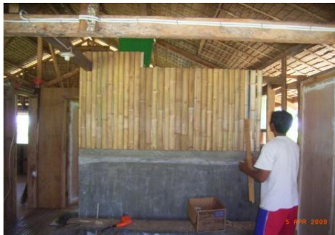
Walling up the T&B. Note aux water tank in green.
