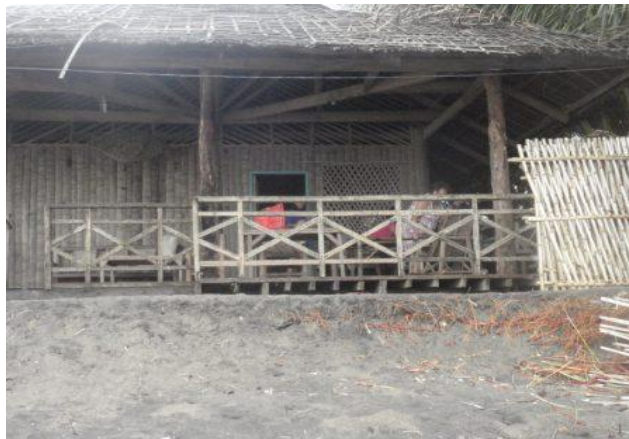
The sea has eaten the shoreline to almost the patio.
