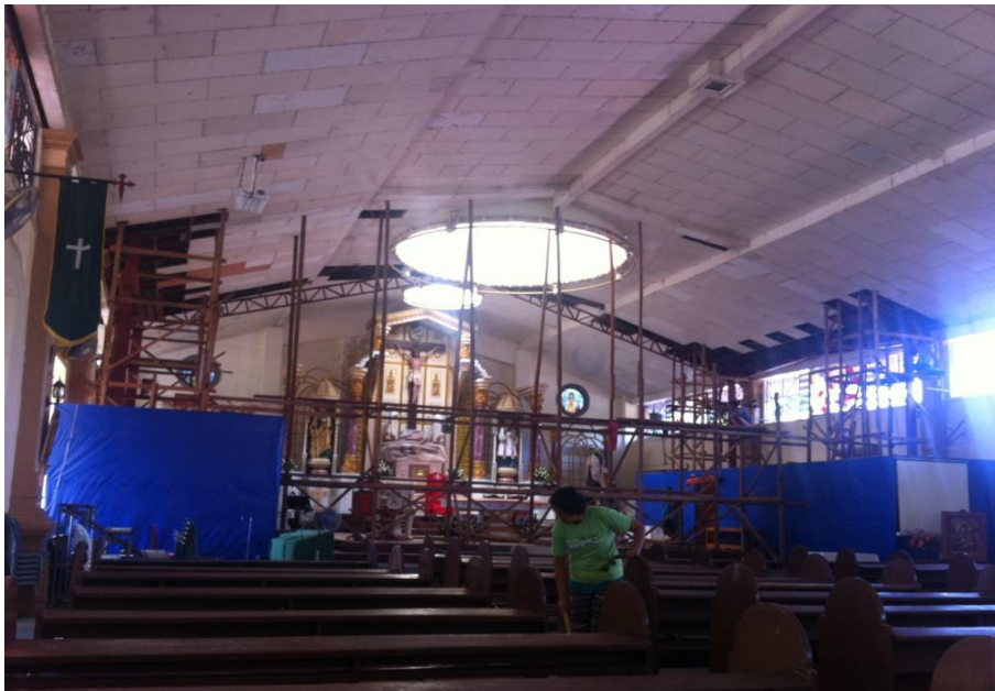
Scaffolding for assembly of second steel beam
