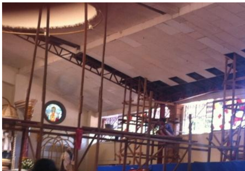
First steel beam which eventually will be covered
