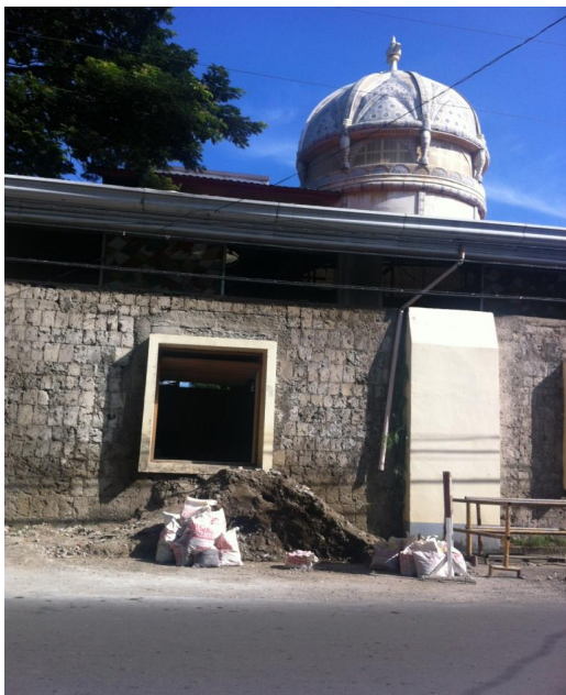
Strengthening of wall
