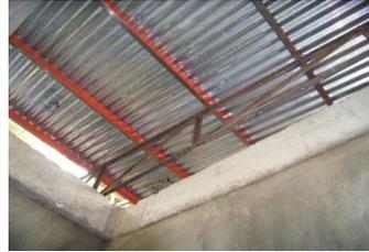
Yes, so true. When we built the house extension six years ago, we used concrete hollow blocks, concrete beams & steel for the roof trusses, as shown on left.
