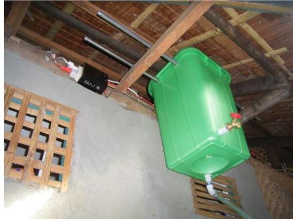
I calculated the weight of the water-filled tank and it came to about my weight, so I did a number of pull-ups on each of the roof rafters and they didn't even budge: therefore, no need for any fancy platform or supporting structure.
